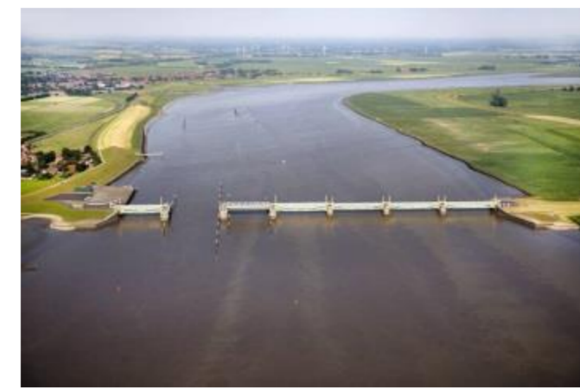
Fig. 2: Storm surge barrier near Gandersum in the river Ems (source: BAW)
