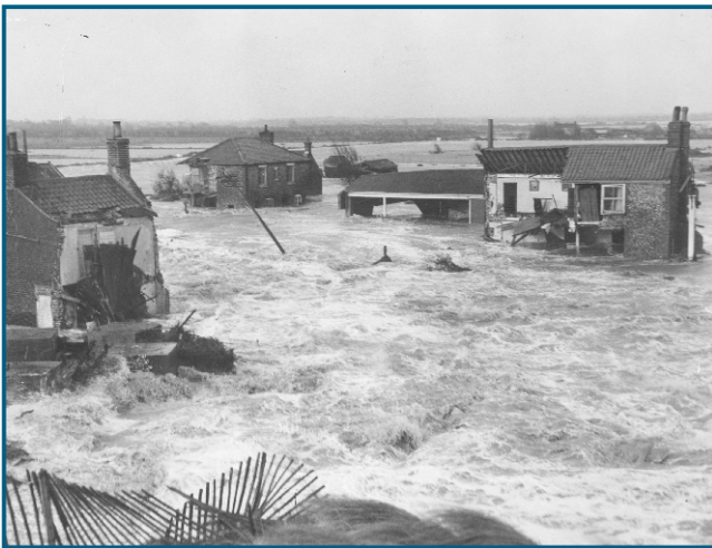
Flooding on the east coast of England during a storm surge in 1953.
