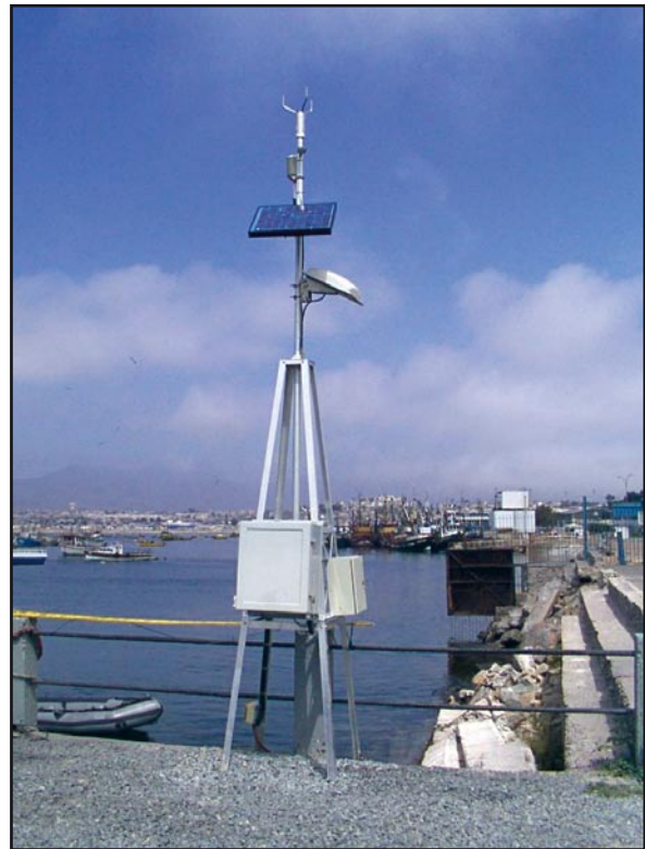
Figure 2. Sea level station configuration.
